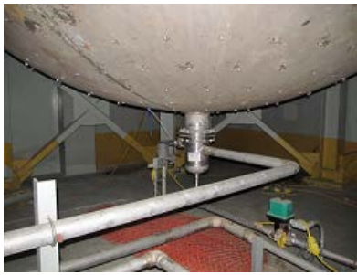
Figure 4 The bottom of the CCT-1 showing valves and pipes reducing workspace (view #1).
